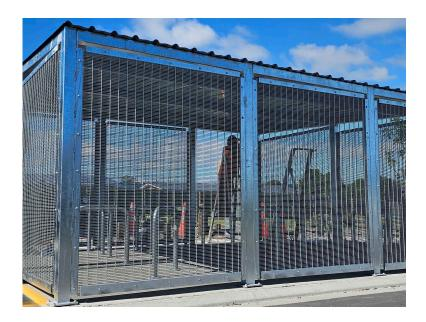
of this bike cage is to protect a wide range of bikes, from children's bikes to E-bikes, from both theft and harsh weather conditions. After thorough consultation with the client and focus on the end user, Hampden produced shop drawings which were later approved for our inhouse fabrication team and the modular system was then prepared for installation and completed in December 2023.
